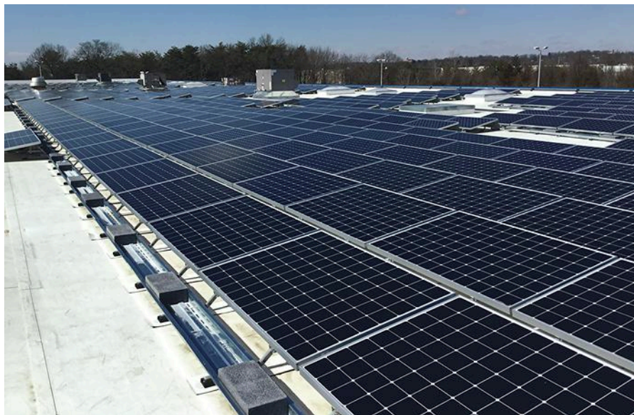
The 925 SunPower solar modules on a Panel Claw support system complete a 302 kW production capacity.
